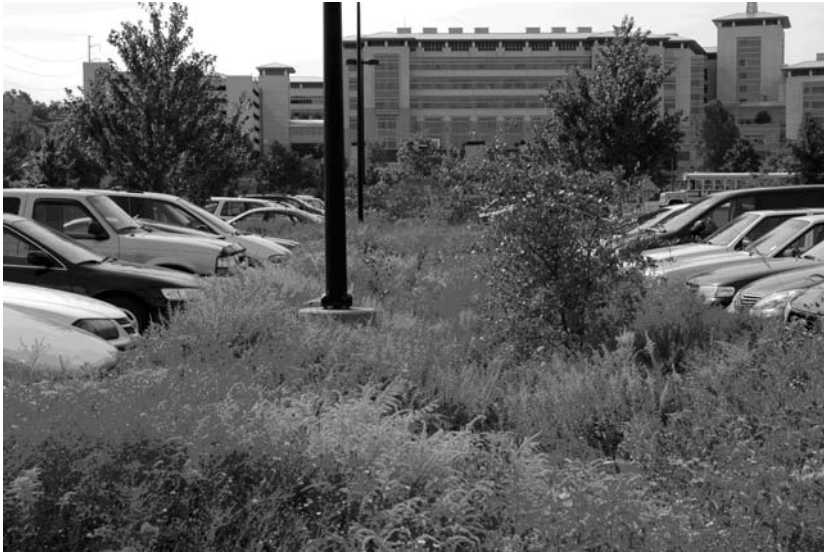
Figure 4.23c Bioswales at Anita B. Gorman Conservation Discovery Center, Kansas City
