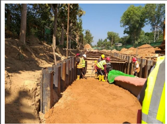
Figure 6.2-1 Earth Retaining Construction
