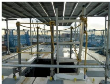
Figure 3.5-4 Fall Prevention at the Opening
