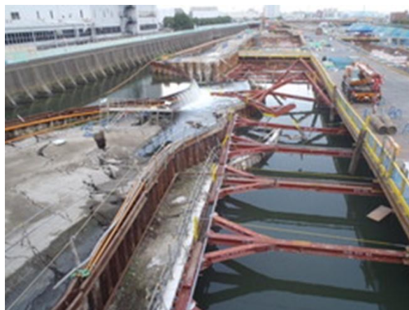
Figure 6.3-1 Temporary Cofferdam
