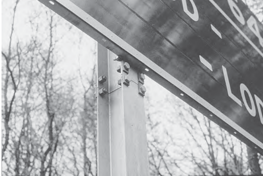
FIGURE 7.31 Commercially available hinge plates by Transpo Industries.
