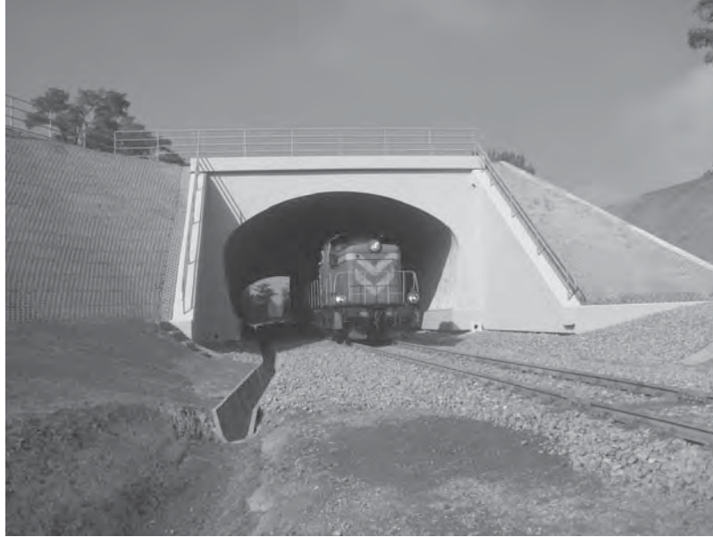
FIGURE 5.43 Corrugated steel culvert being used as a railroad overpass. (Photograph with permission of Viacon, Polska)
