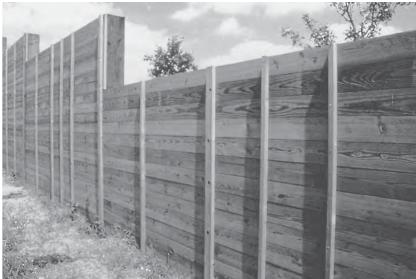
FIGURE 9.3 Timber noise barrier with tongue-in-groove construction, stepped in height.
