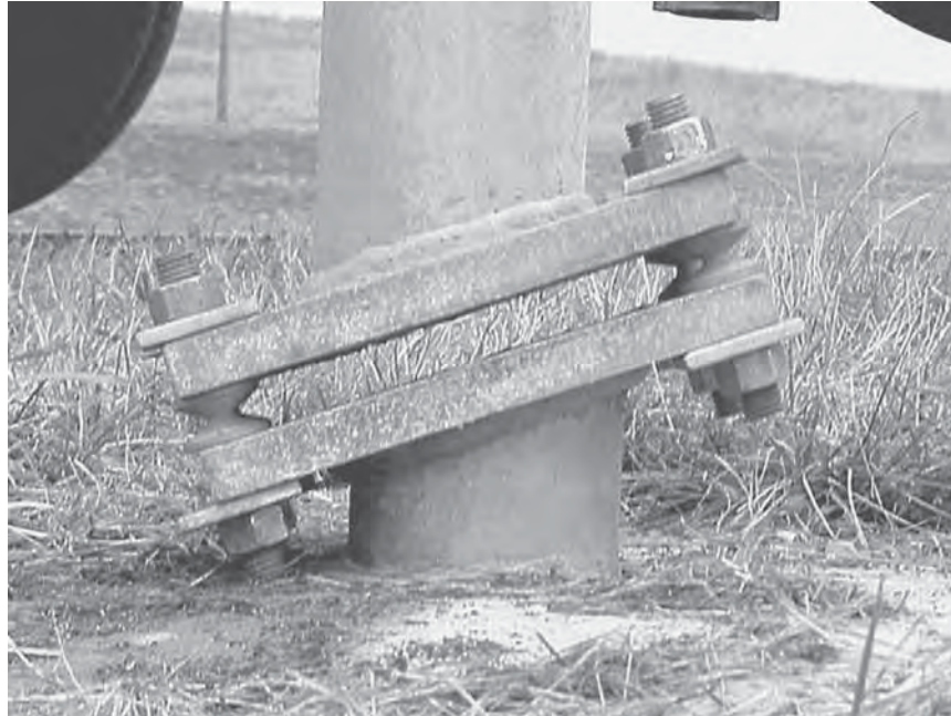
FIGURE 7.21 Frangible-coupling sign support.
