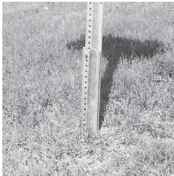
FIGURE 7.10 Improper splice of U-channel post system.
