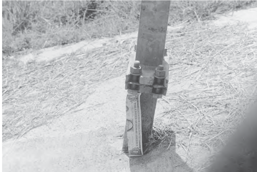
FIGURE 7.37 Improper installation of slip base anchor piece.
