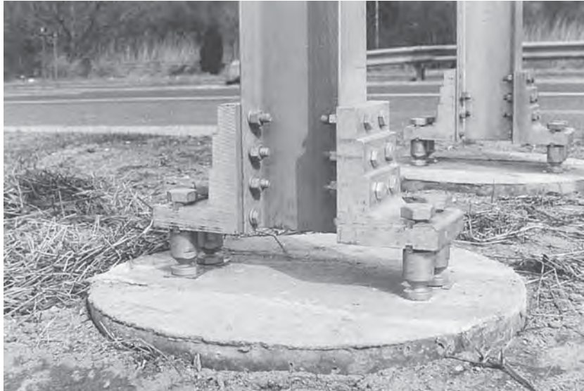
FIGURE 7.28 Base with load concentration couplers.
