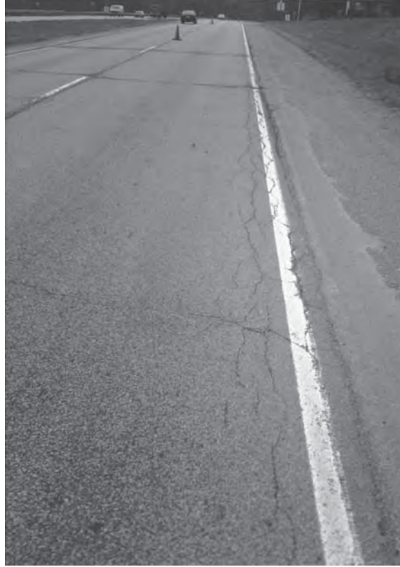
FIGURE 3.40 Example of edge cracking in flexible pavement.
