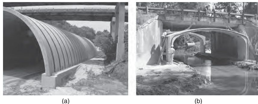
FIGURE 5.42 Two examples of reinforced concrete arch structures being used as bridge replacements. (Photographs with permission of Contech Bridge Solutions, Inc.)
