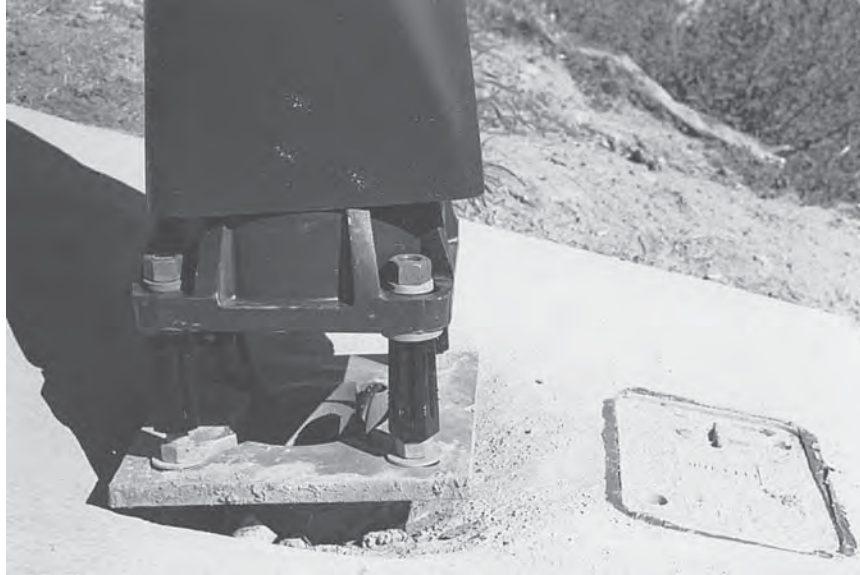
FIGURE 7.74 Frangible-coupling luminaire support.
