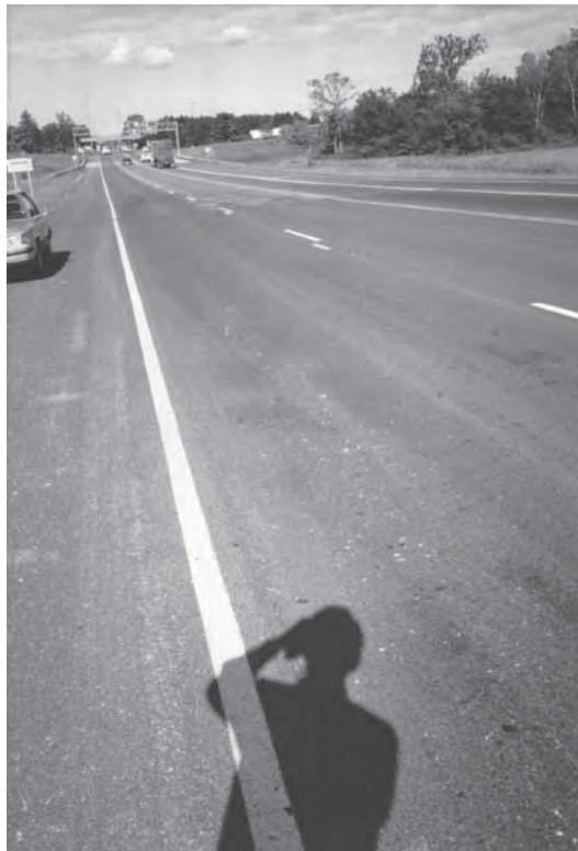
FIGURE 3.32 Example of bleeding in flexible pavement.
