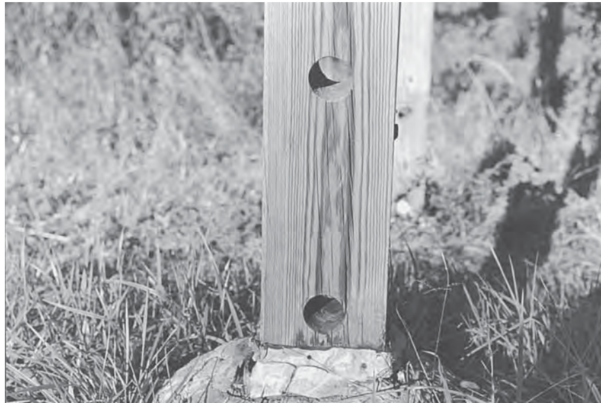
FIGURE 7.46 Weakened wooden post for multiple supports.
