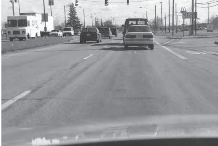
FIGURE 3.34 Example of rutting in flexible pavement.
