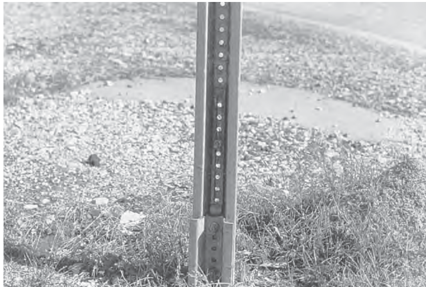
FIGURE 7.6 Example of breakaway single sign support.
