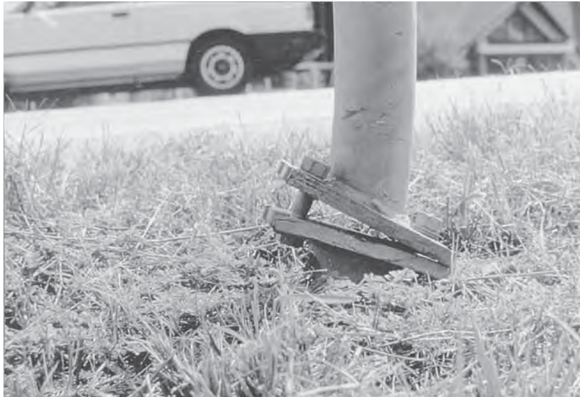
FIGURE 7.17 Loose slip base caused by vibration.
