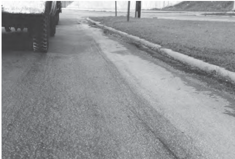
FIGURE 3.35 Example of corrugations in flexible pavement.
