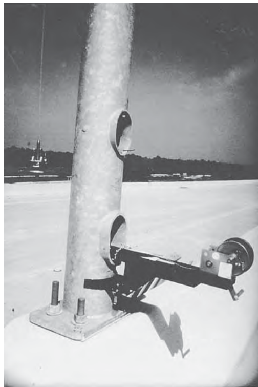
FIGURE 7.60 Lowering device manufactured by ITS Products Inc.
