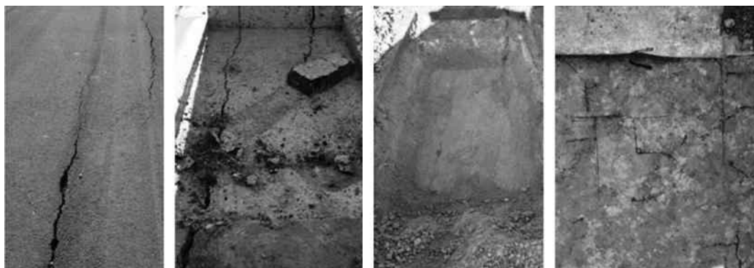
Figure 15.9 Shrinkage cracking owing to subgrade shrinkage; cracks shown on each layer and on the surface of the subgrade.
