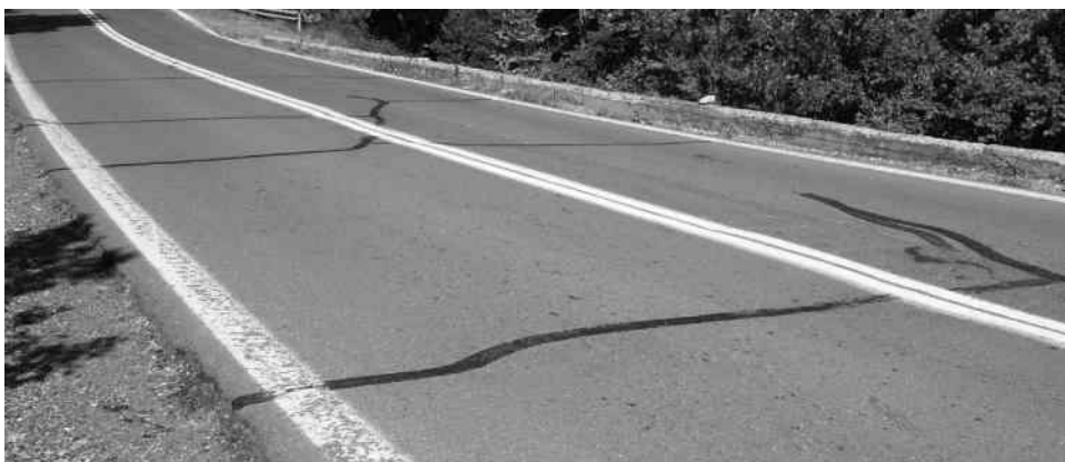
Figure 15.8 Shrinkage cracking, block patterned.
