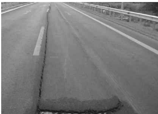
Figure 15.11 Slippage of asphalt overlay over a geotextile.
