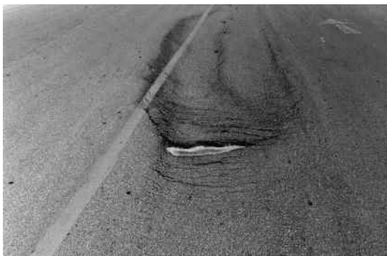
Figure 15.7 Slippage cracking. (From Asphalt Institute, Asphalt in Pavement Preservation and Maintenance , Manual Series No. 16 [MS-16], 4th Edition, Lexington, US: Asphalt Institute, 2009. With permission.)
