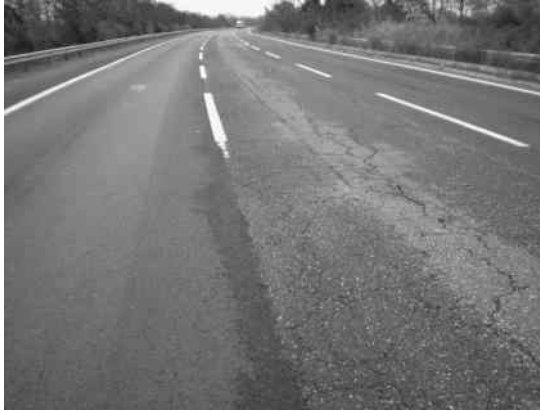
Figure 15.5 Reflective cracking initiated over an old paving joint in a flexible pavement.
