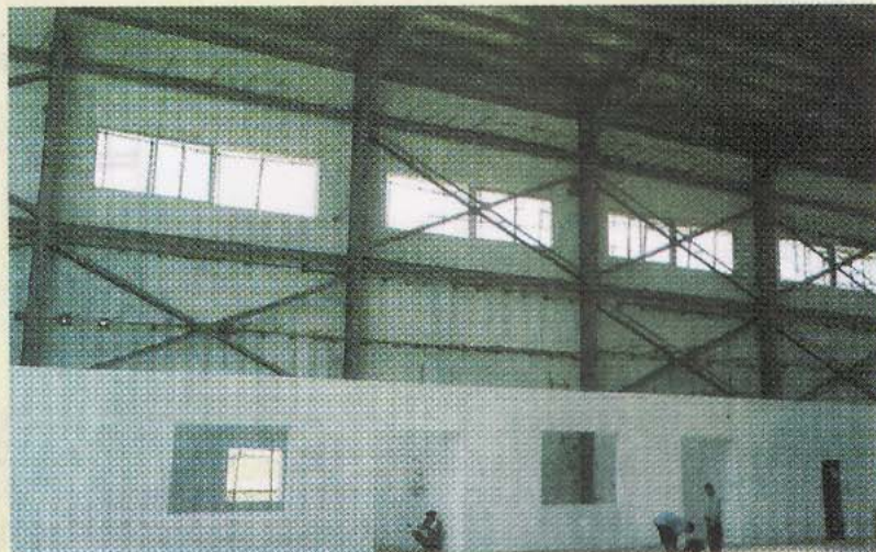
Column diagonal bracing
