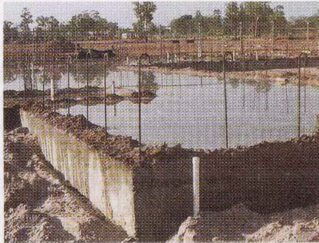
Concrete slab cured by ponding
