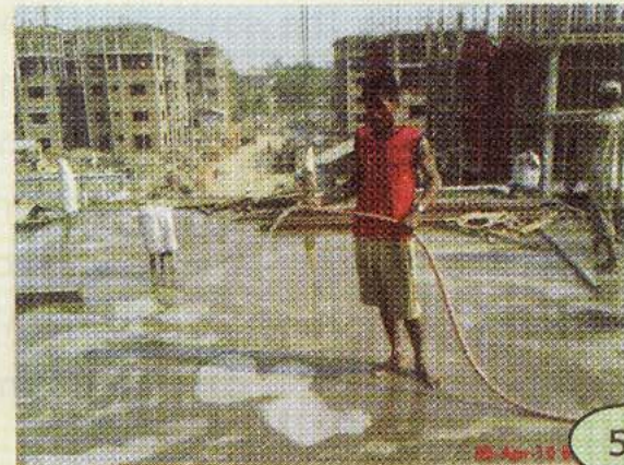
Spraying water to cure the slab
