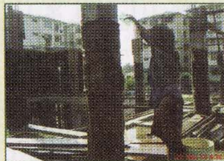
Wetting the gunny wrapped around the column
