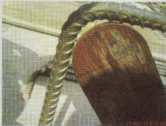
Checking the radius of a 90° hook
